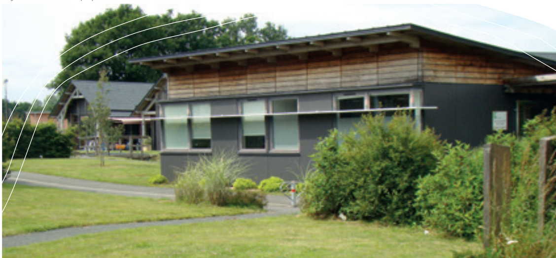
Foyer de Vie du Cœur (44) | Ad Hoc Architecture | © MANA
